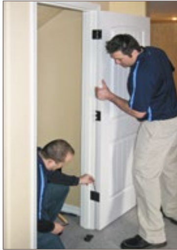
New doors and hardware are installed
