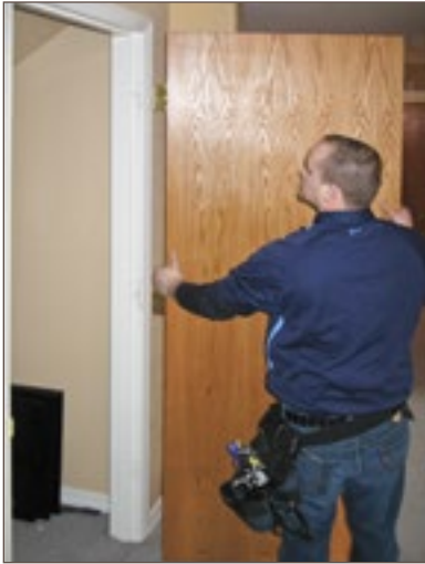
Your existing doors are removed
